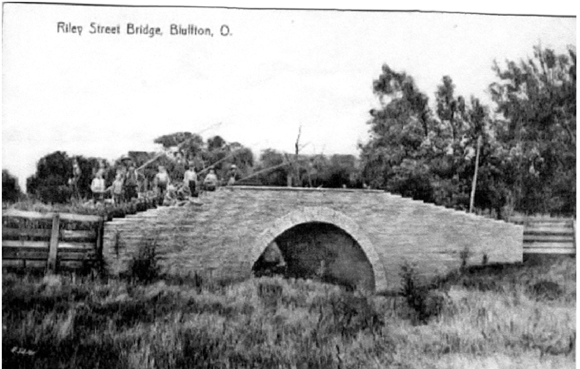
Arch Bridge on Riley Street
