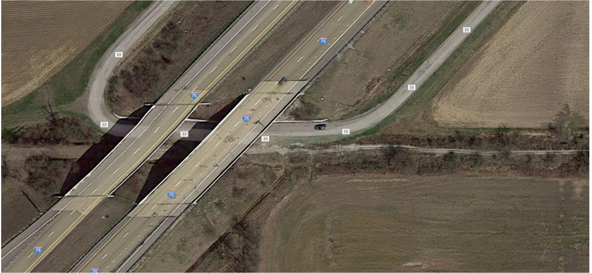
Interstate 75 bridges over abandoned Akron, Canton and Youngtown Railroad
