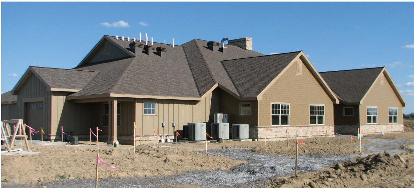
This is a view from the back of House B. The stone pathway shows how a sidewalk will connect both houses together, making it easy for elders and guests to visit one another. The curbs of Willow Ridge Court have been poured and sidewalks are nearly complete. The exterior paint on both houses is almost finished.
