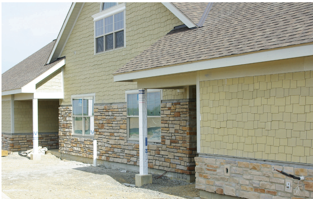
A view of the south side of House B.
