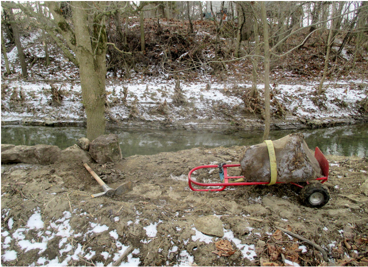
The red cart at rest: David has single-handedly engineered the move of over 30 tons of rocks to separate the quarry wetland from Cranberry Run. The creek was channelized in the 1950s which allowed sediment-laden floodwaters to fill the quarry that once was a popular fishing spot. In order to prevent the vital wetland from completely filling in and to allow visitors to observe creek and wetland life side-by-side, David has reconstructed the lost bank between the two bodies of water.
