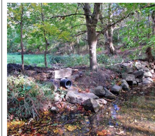
Engineer David Seitz is in the process of developing a system that will allow Cranberry Run to supply water to the quarry wetland while preventing increased siltation during flood events. See details on the back of this newsletter.
